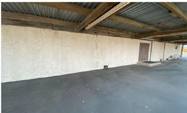
East Wall – Before
