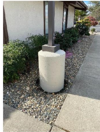
Finished Light Post
