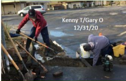
Gary Okamoto Kenny Teranishi Lloyd Okimura Ben Kusaka all helped to replace the stop drain value on 12/31/20
