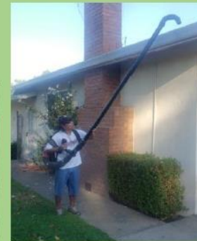
Gary & Kenny working on drain value replacement.
