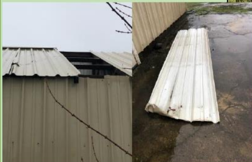
Tool shed roof
